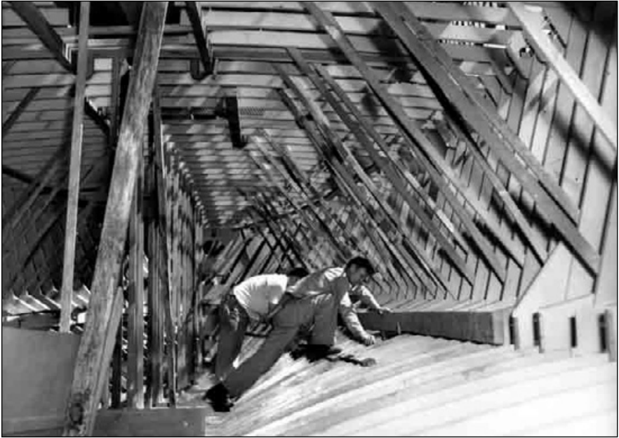
11. The construction of fast, motor torpedo boats out of wood for the US Navy in the Second World War. They were built undercover, of pre-fabricated sections. Production techniques for seemingly old products and materials were changing just as they were in 'new' industries.
