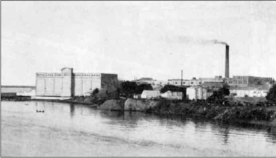
23. The Frigorífico Anglo, Fray Bentos, Uruguay, in the interwar years, showing the chilled meat warehouse (cold store) on the water's edge. A plant had existed here since the 1860s, first making Liebig's Extract of Beef. The plant remained in operation until the 1970s and is now preserved as a Museum of the Industrial Revolution.
