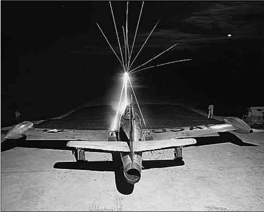
13. The 0.5 inch guns of a Republic F-24 Thunderjet fighter-bomber are tested by its maintenance crew in Korea, 1952. Air forces have typically had many more maintenance personnel than pilots.
